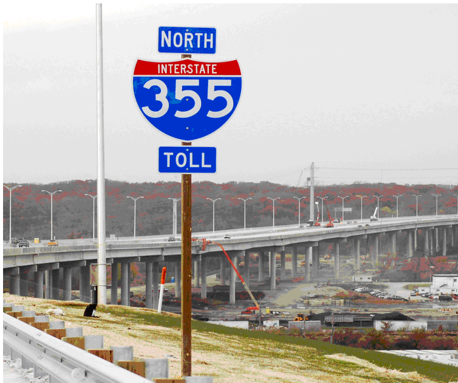
Northbound view of the Des Plaines River Valley Bridge
