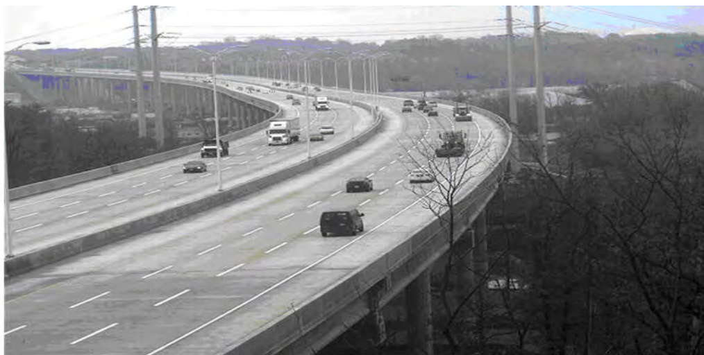
Des Plaines River Valley Bridge
