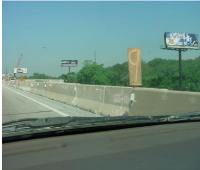
Unclear Construction Entrance
