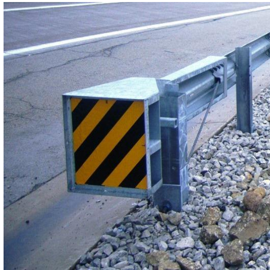
Figure 10.3.1b Traffic Barrier Terminal Type T1 (Special) - With Modified Gutter
