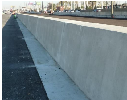
Figure 13.3 Concrete Barrier Double Face
