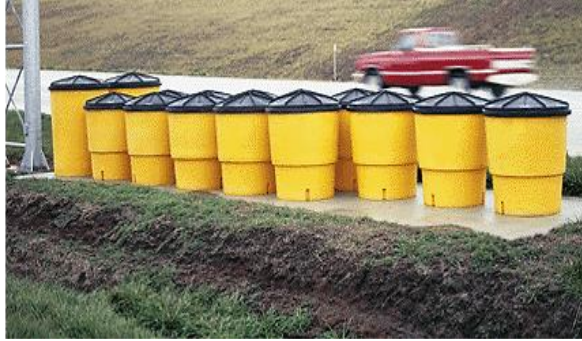
Figure 11.2 Sand Module Impact Attenuator
