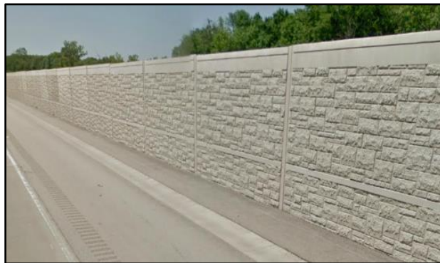
Figure 3.8b Noise Abatement Wall Attached to Parapet (Structures)
