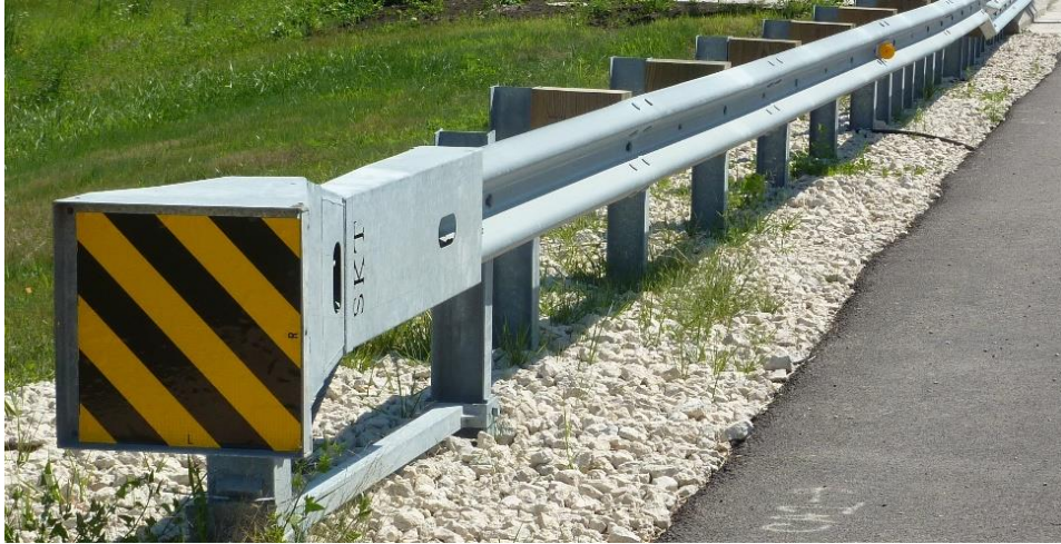
Figure 10.3.2a Traffic Barrier Terminal Type T1-A (Special)
