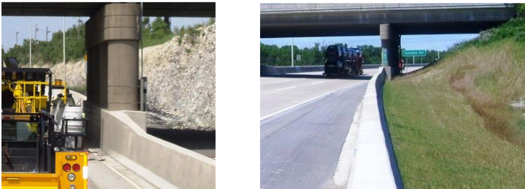
Figure 13.2a Concrete Shoulder Barrier Transition
