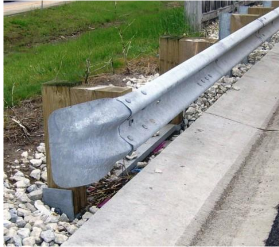
Figure 10.5.1b Traffic Barrier Terminal Type T2 – Without Gutter
