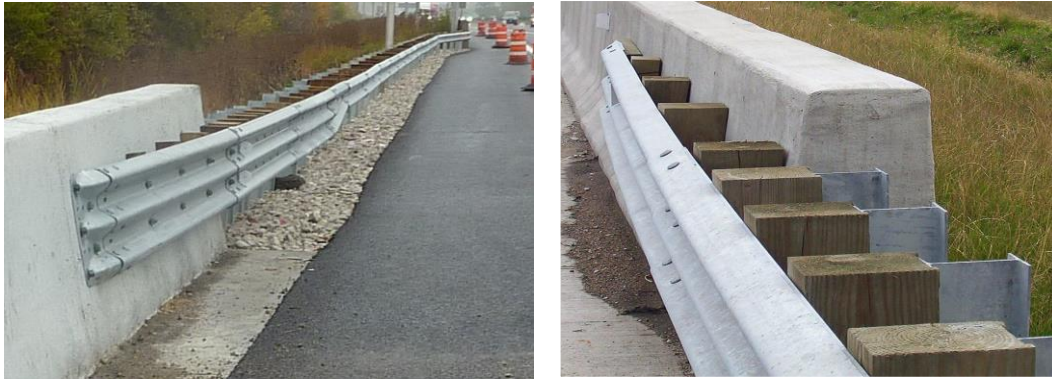
Figure 10.6.2 Traffic Barrier Terminal Type T6B
