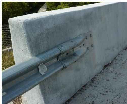
Figure 10.4.2 Traffic Barrier Terminal Type T10
