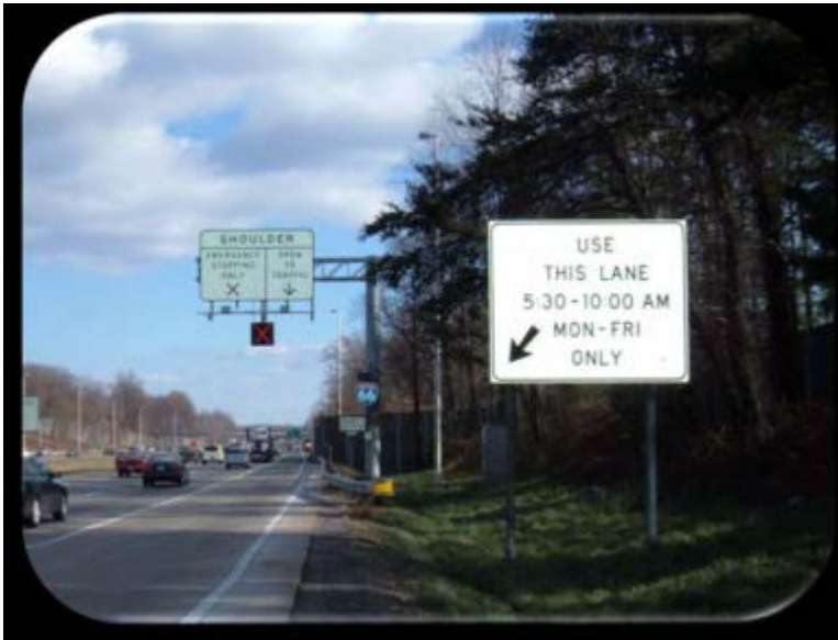
Source: FHWA I-66 in Virginia
