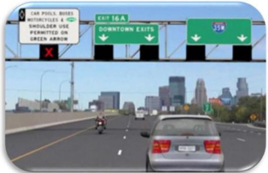
Source: FHWA MnDOT
