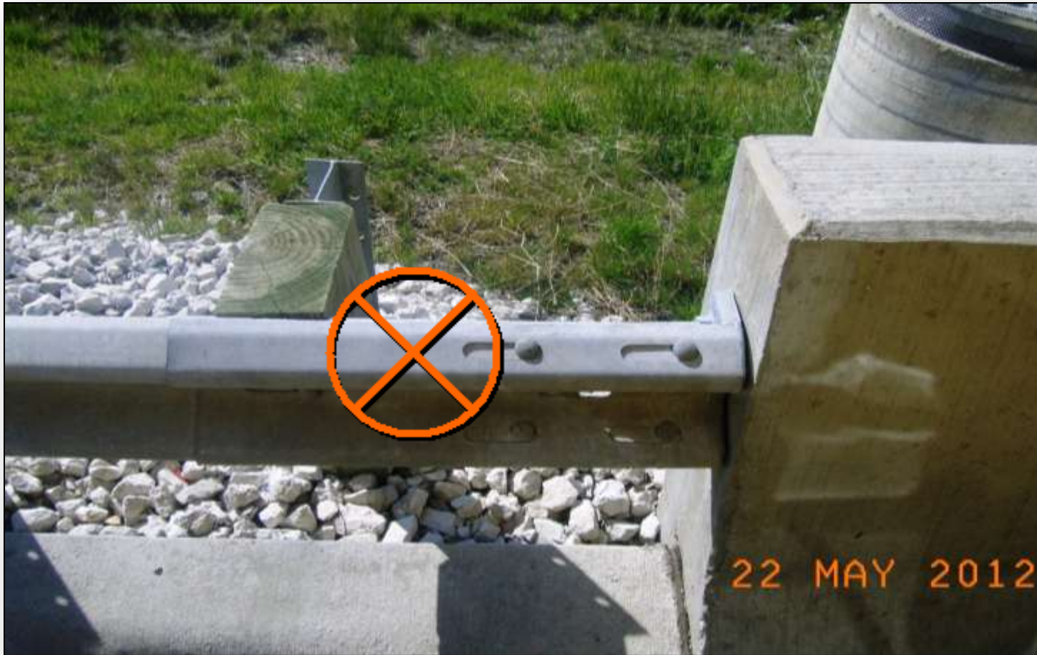
Plate G was placed over the rail element.
