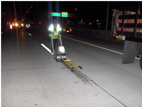
Figure 10. Tape laid and cut with tape cart.
