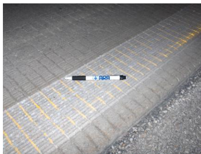
Figure 6. Edge line groove ready for pavement marking.
