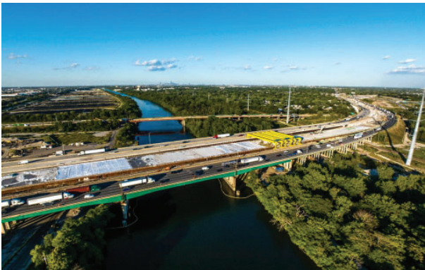
I-294 Southbound Mile Long Bridge Project near Willow Springs.
