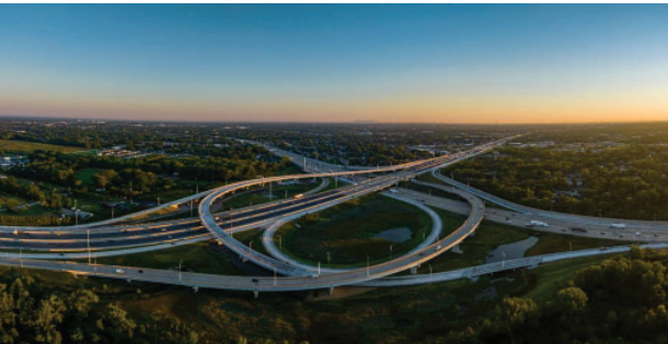
Completed I-294/I-57 Interchange near Harvey, Markham.
