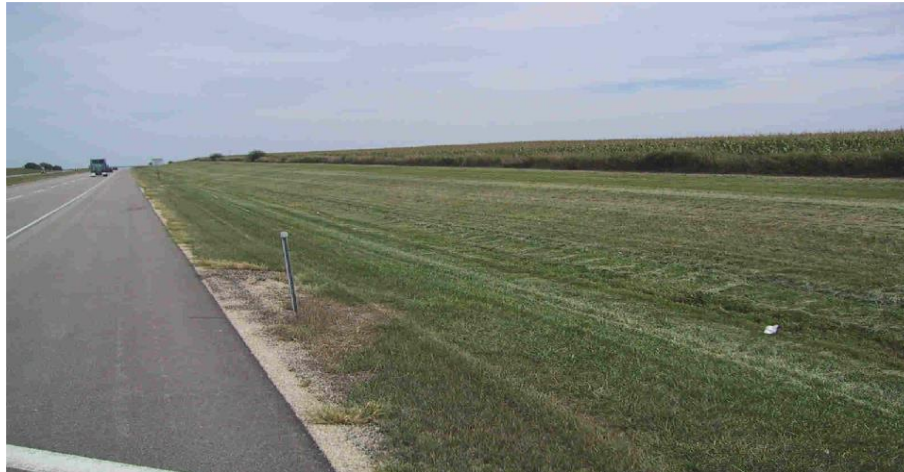
Example: less desirable conventional backslope turf mowing practice
