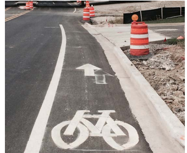
New bike lane installed as part of Elgin O'Hare Expressway construction.
