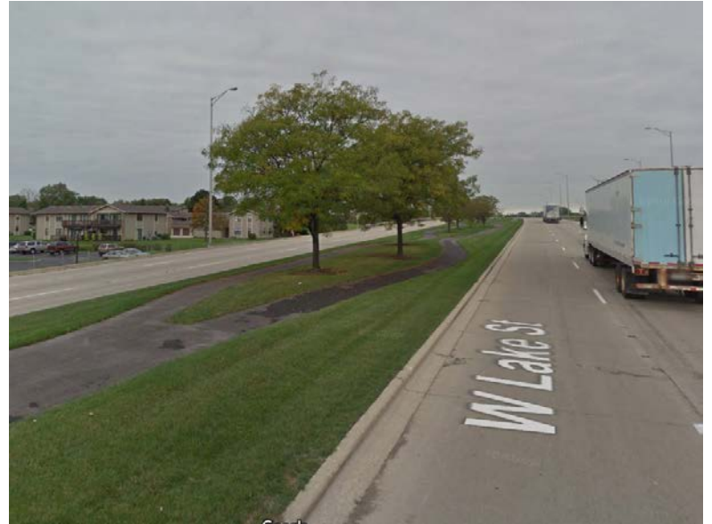
New bike lane installed on US 20 at IL 390
