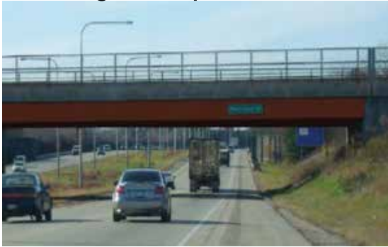
Steel girder paint
