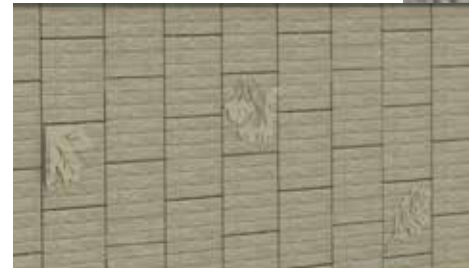
Leaf formliner on retaining walls
