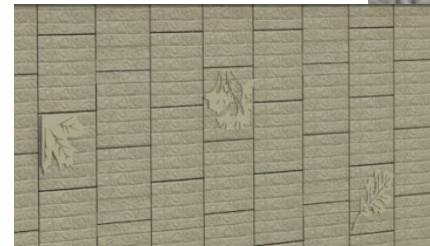
Leaf formliner on retaining walls
