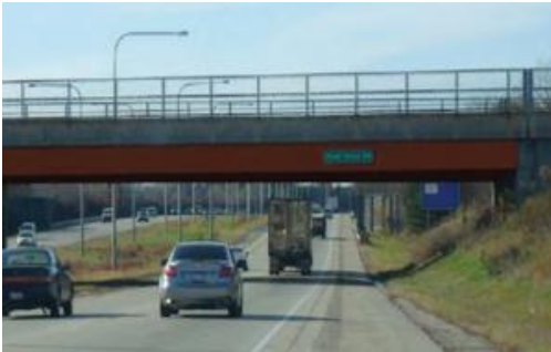
Steel girder paint
